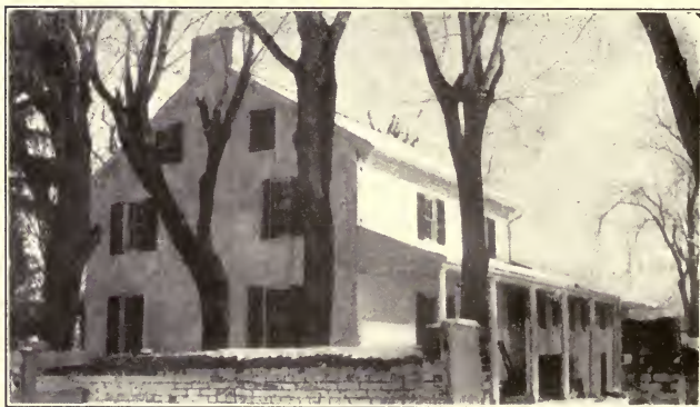
Old Brick Wall with Moulded Cap
